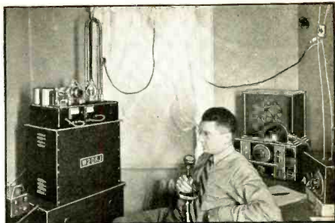
The Operating Shack at W2DKJ—The 5-40-100 Transmitter with its "power-supply" is shown on the small table, directly in front of the author. The Modulator and National Midget Oscilloscope are shown to the left. The low-impedance cables draped above the author's head run to the antenna relay which is on the other side of the window shade. The National NC-100X receiver is used on the ten and other lower frequency bands while for five meter operation a National 1-10 receiver has proved to be most satisfactory, after many other types of receivers were tested. It will be observed that Mr. Lynch favors a Crystal Microphone.
