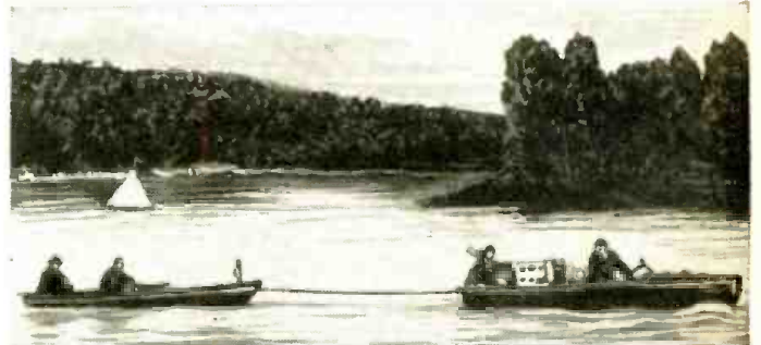
Fig. 1—To determine the variation of the field strength with distance the receiver was located in a small motor-boat which towed a rowboat with the transmitter aboard.
